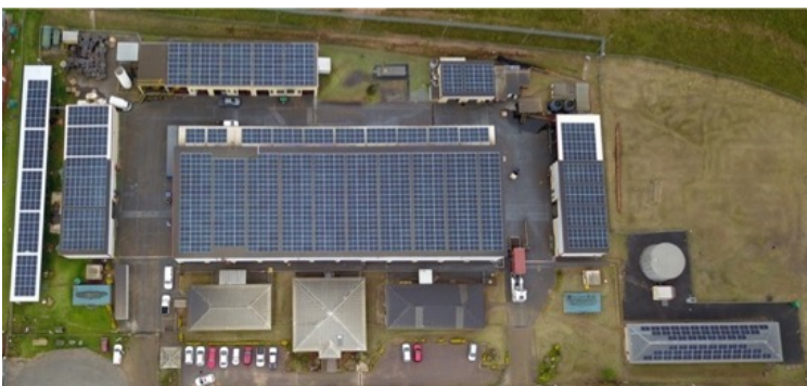
Fig 15. Solar panels covering 90% of Shu Powders roof space to generate electricity.
