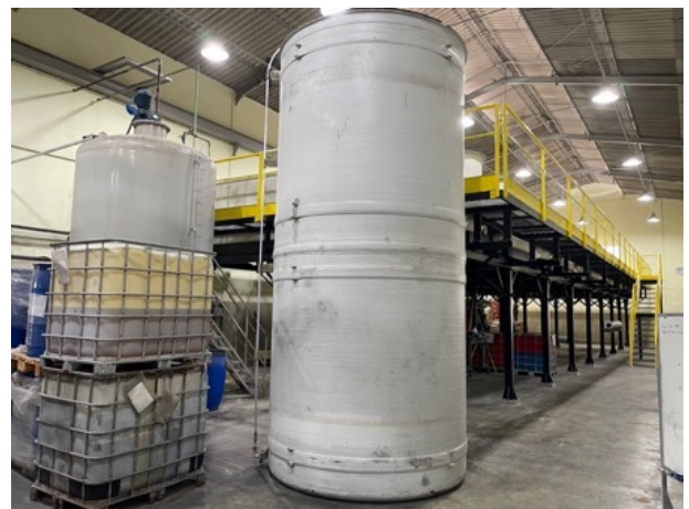
Fig 12c, Incasa Co refinery: Installation nearing completion of the new Co:Ni separation line mid 2022.
