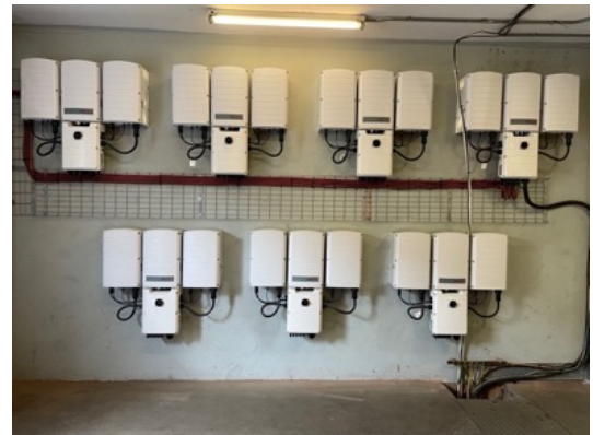
Fig 12c, Solar Panel Inverters: Seven inverters installed for 630 kW.
