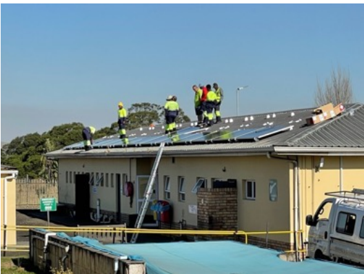
Fig 12a,b, Solar Panels: Installation in 09-2024
