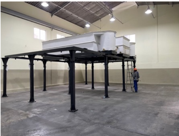
Fig 12c, Incasa Co refinery: Installation starting of the new Co:Ni separation line using solvent extraction technology early 2022.
