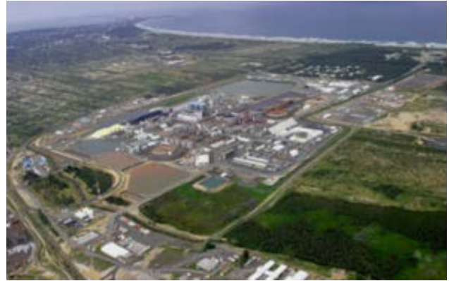
Pic 6b, Ambatovy: The facilities in Madagascar are owned by Sherritt, Sumitomo, Kores.
