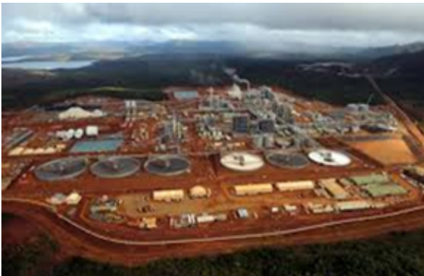
Pic 8a, Goro: The facilities in New Caledonia are owned and operated by Vale INCO.
