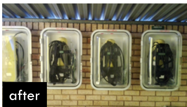
Fig 9 a,b : Air supply cylinders for ammonia emergency alarm teams have been refurbished and prepared for easy access.
